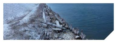
Failed timber wall at toe of steep bluff. A revetment or seawall would be suitable protection for this shoreline.
