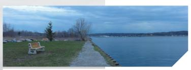
East end of the study area. The Steel Sheet Pile (SSP) wall appears to be in reasonable condition. Water depth is most likely deep (18 ft estimate). This used to be a quay wall for ships to load. A floating dock could be used to improve accessibility for boats. A detailed inspection was beyond the scope of this study.
