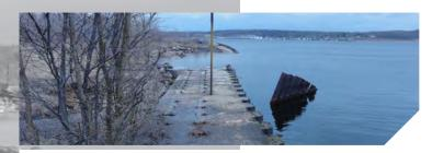
The SSP wall starts to fail a couple hundred meters along the wall. There are signs of undermining and the concrete has detached from the SSP. Some of the slabs have started to shift.
