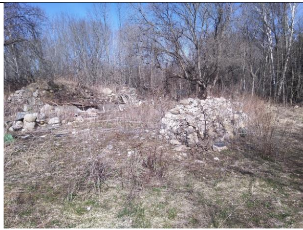
IMAGE 11 FORMER BARN FOUNDATION AND WALL
