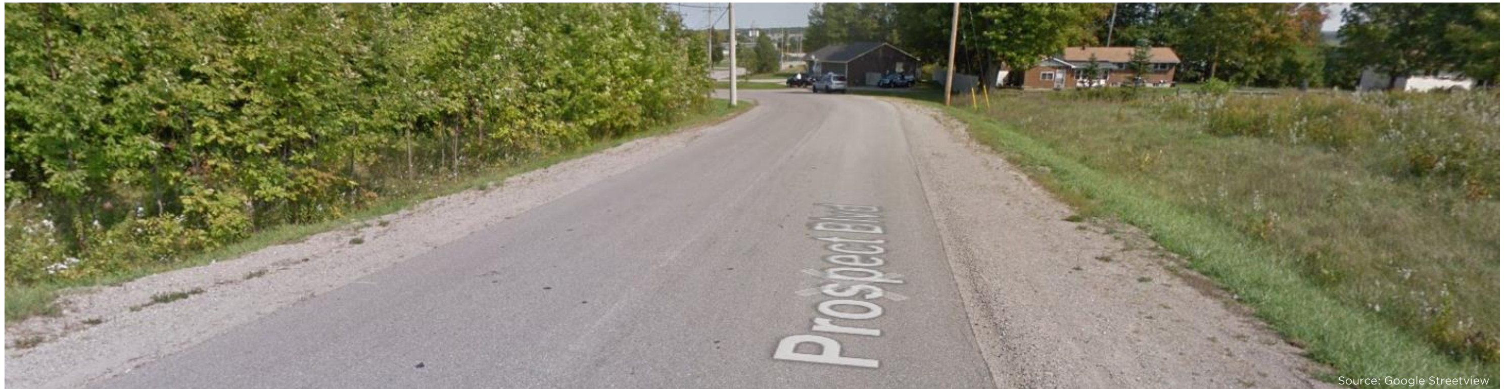
Looking east along Prospect Boulevard from site access
