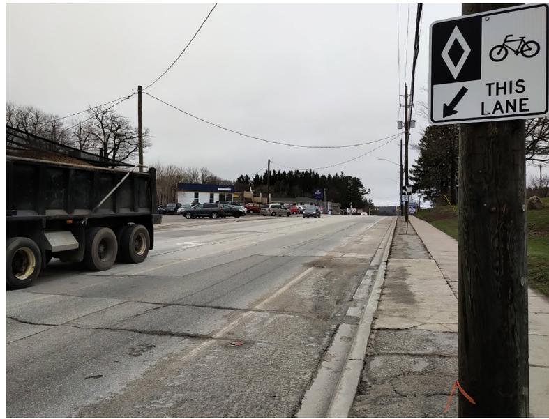
**Figure 2.9** The newly dedicated bike lanes on Yonge Street have no distinguishing design features from the adjacent general traffic lanes besides the signage, particularly in the winter when the paint markings disappear due to winter maintenance.
